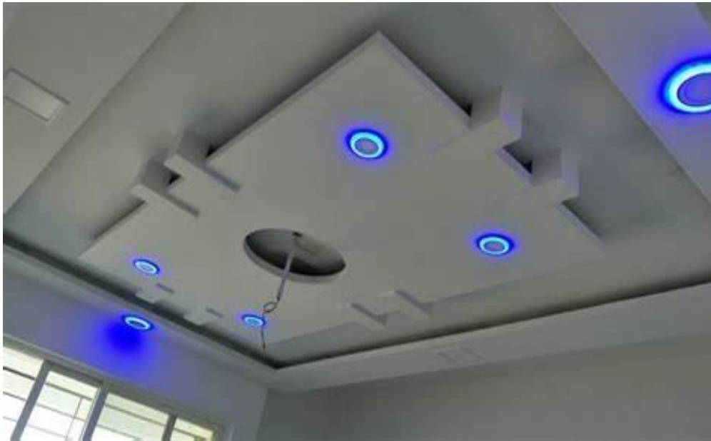
Fig. 2. POP ceiling finishing Source: [7]
