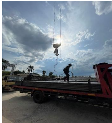
Fig. 2. Material mobilization from stockyard to work site
