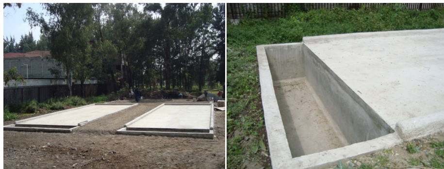
Figure 1. Concrete slabs and pits designed.
