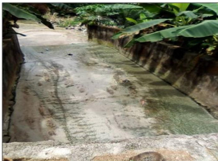
Fig. 4. A wastewater channel in an industrial facility
