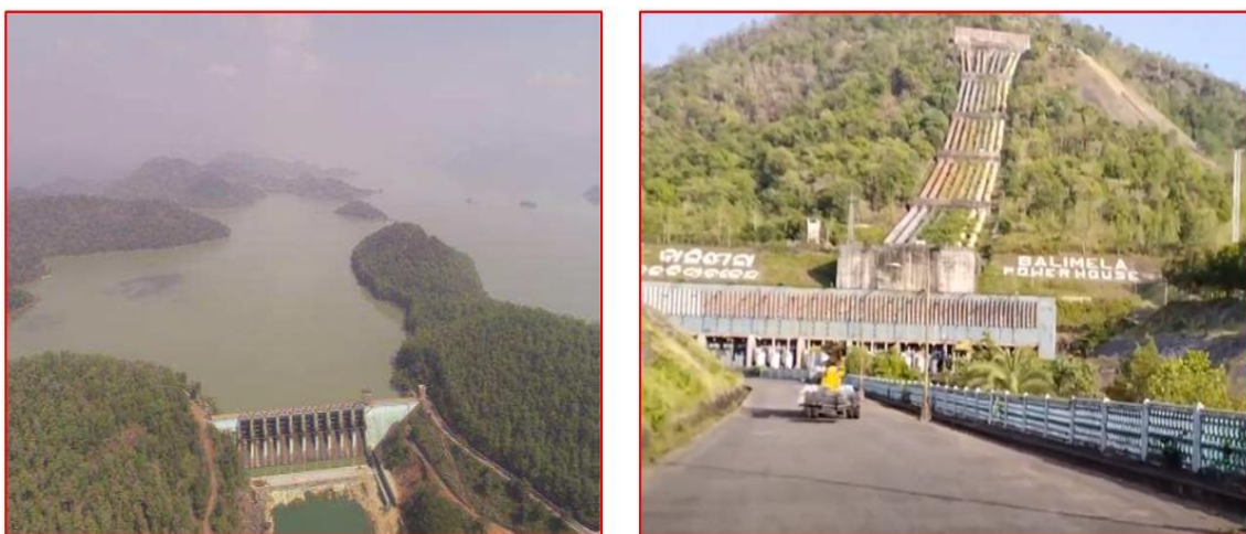
Fig. 2. Balimela Power House and Chittrakonda dam on the Sileru River; Odisha
