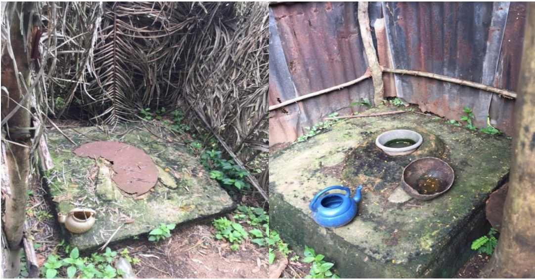
Plate 3. Pit latrines built with thatched leaves (C) and roofing sheet (D) frames
