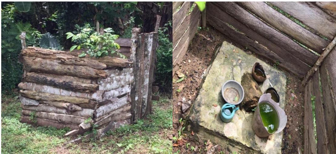
Plate 2. Exterior (A) and interior (B) of wooden frame pit latrine
