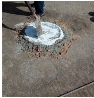
(b) Cement and recycled glass powder added to fine
