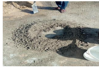
(f) Water added to the mixture of fine aggregate, cement, recycled glass powder, coarse aggregate and shells of palm kernel
