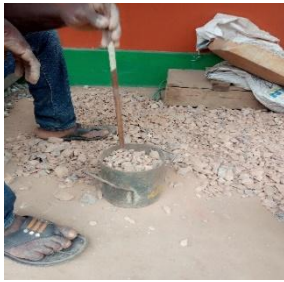
(d) Tamping rod permitted to fall easily from a height of 50mm above the surface of the aggregate
